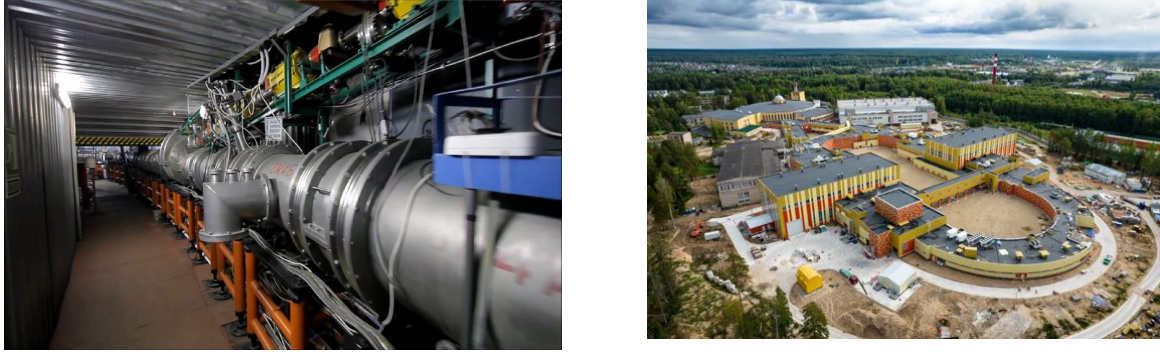
Figure 2: (Left) Nuclotron (Left). (Right) NICA aerial view, April 2022.
