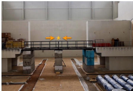
Figure 27: SPD experimental hall under construction
